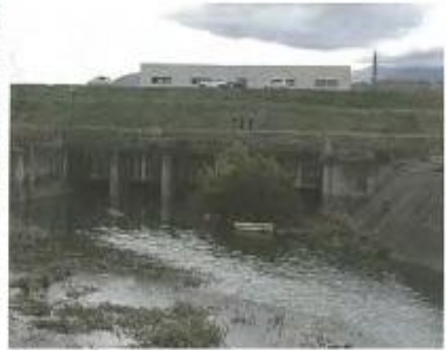
Figure 22a. Sediment deposition from apron Figure 22b. Vegetation in front of gates To box culvert
