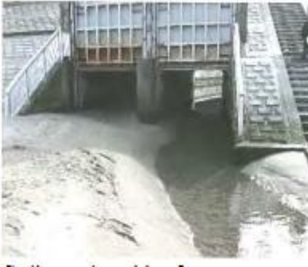
Figure 22a. Sediment deposition from apron Figure 22b. Vegetation in front of gates To box culvert
