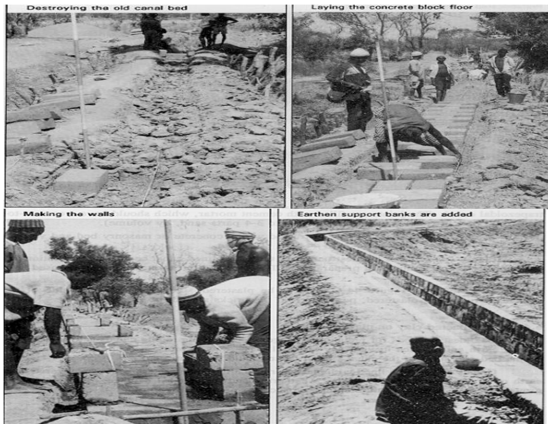
Figure 24. Repairing concrete, brick and stone structures
